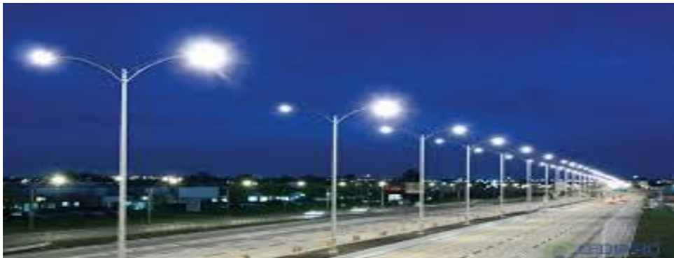
Fig.1. Street lighting using LEDs vs. old generation street lighting
